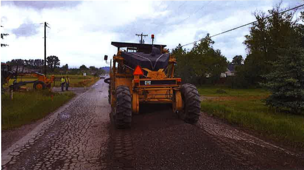
Bonner County equipment pulverizing and mixing the asphalt on Main St.
