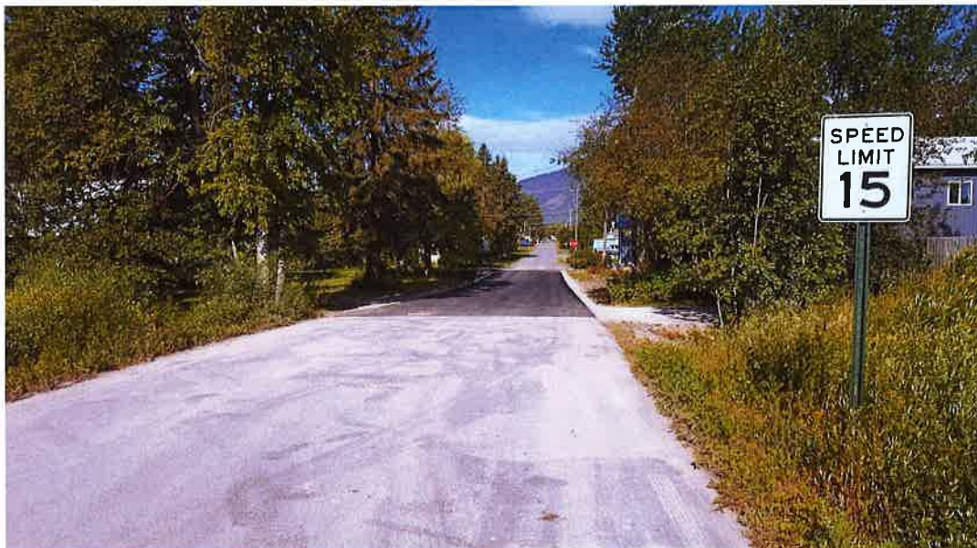
E. 2 nd Avenue – pavement and signage in place.
